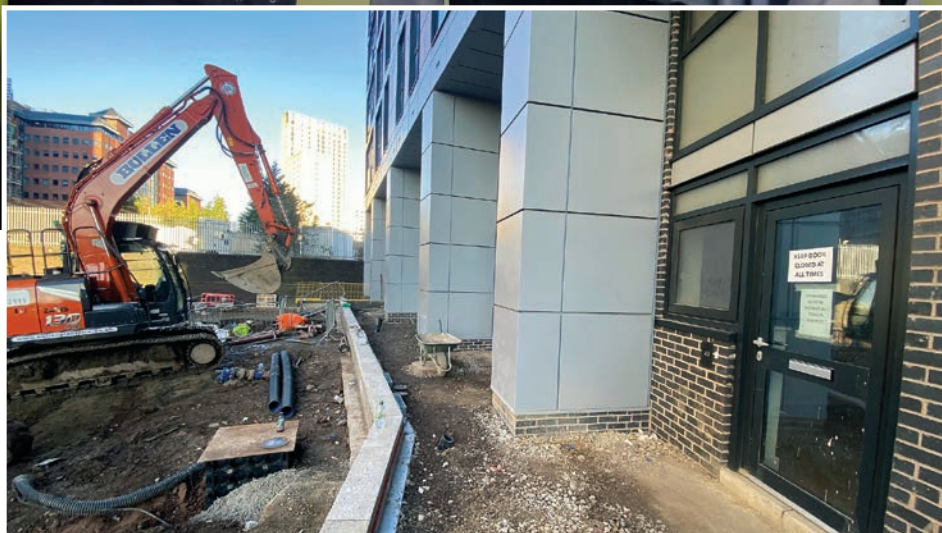
Members of Recom's passive fire protection team on site. "It requires a certain level of competency to make a building fit for purpose," says Jason McKnight
